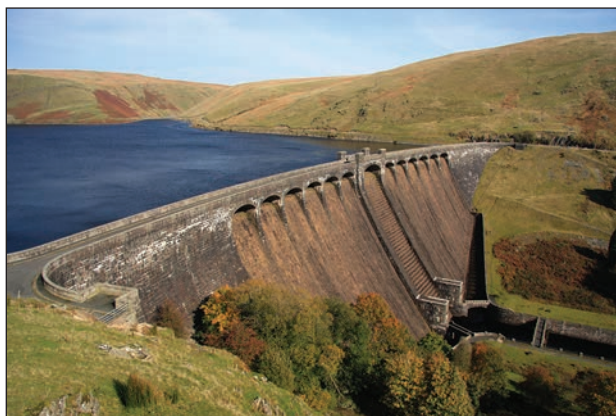
Reservoir and dam in Wales
