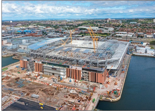
Building the new Everton Football Club stadium
